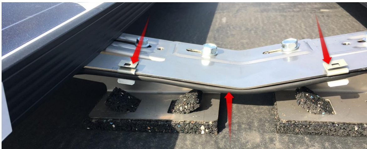
Figure 15: Correctly attached DC cabling
